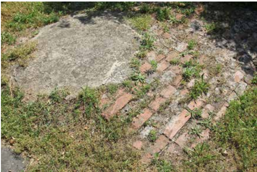
Constructed into the side of a hill (photographed on November 8, 2015, above, and June 19, 2016, left), red bricks form the vault's convex roof. Cement now covers the vault entrance, where the capstone may have been.
